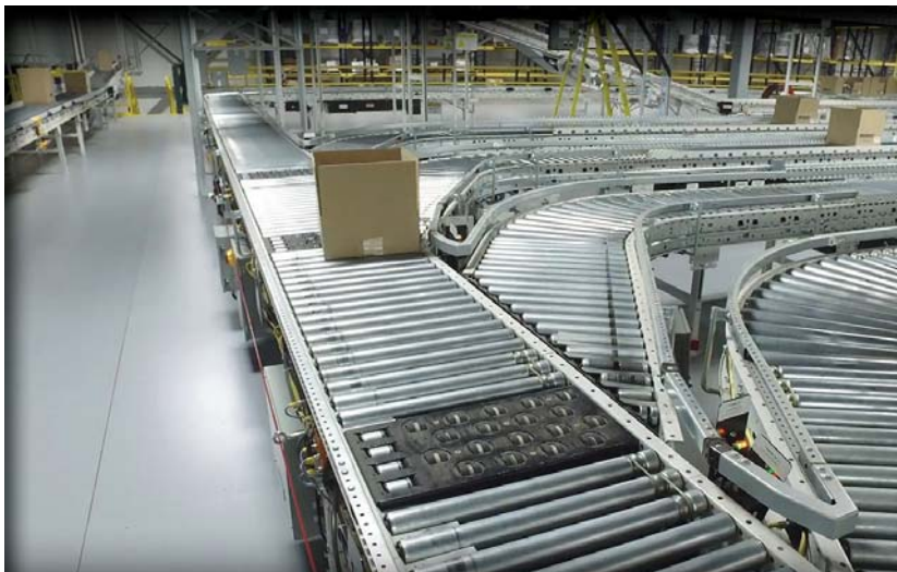
Werner Electric uses Tecsyst to power its fulfillment operations.
