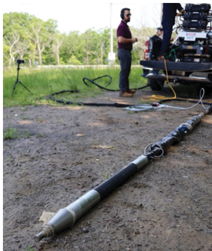
3. GE Vernova’s SPEEDWORM technology installs conduit and cables for underground distribution power lines in a single step, mimicking the movement of earthworms and tree roots to install 1,000 feet of cable and conduit in about two hours, according to the company. Courtesy: GE Vernova
