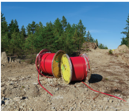
2. Cables installed in buried conduit are shielded from wind, ice, vegetation, vehicles, and ignition sources—trading upfront construction cost for decades of reduced outages and avoided wildfire liability. Courtesy: VidEst / Envato Elements
