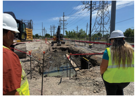
5. Flooding is one of the biggest threats to substation equipment. In Lockport, Louisiana, Entergy crews are building a reinforced flood wall around the Valentine substation, the first of five projects like it planned across the state. Courtesy: Entergy
