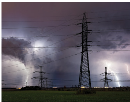
1. Severe weather, including lightning, is a major cause of power outages. Electric utilities and grid operators are using a variety of technologies to harden the power delivery system against extreme weather events. Courtesy: kijeviskymarek / Envato Elements
