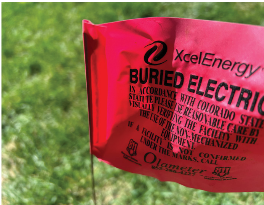
5. Xcel Energy has buried power lines in neighborhoods across its service territory, including in Colorado. The utility uses undergrounding as one of several tools to support the power grid and reduce the risk of wildfires. Source: POWER
