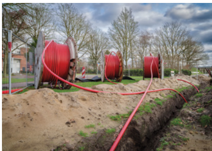
2. Crews install underground conduit for medium-voltage distribution cable—a weather-hardening approach increasingly favored over overhead lines in storm-prone regions. Courtesy: wirestock / Envato Elements
