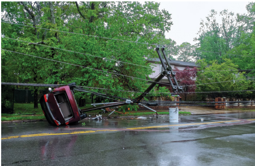
1. A single vehicle impact can topple a pole, drop live conductors into the street, and cut power to an entire neighborhood. Undergrounding removes the target from the roadside. Courtesy: photovs / Envato Elements
