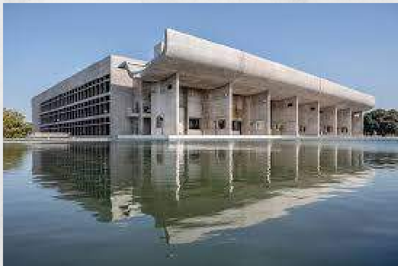
High Court, Chandigarh by Le Corbusier
