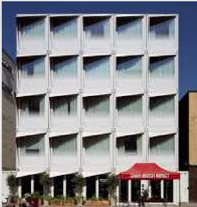
Stow-Away Hotel by Doone Silver Kerr || Made by stacking shipping containers
