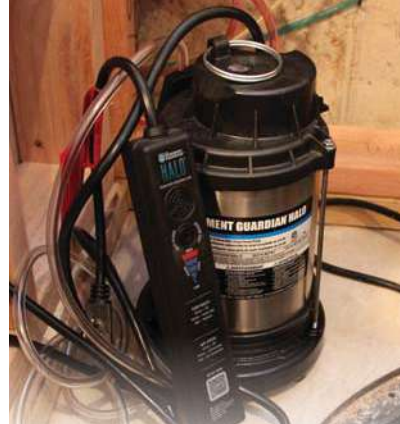
Engineers at Grid Connect found that by measuring current leakage in a sump pump, they could predict pump failure. They worked with pump manufacturer Wayne to develop an app-based monitor for the homeowner. Grid Connect/Wayne
