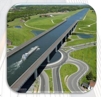
65,000 tons and was progressively launched into place (world record). Beginning of works: 1998 Completion: 2002
