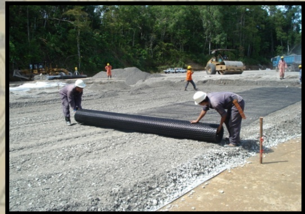
Fig: Application of geosynthetic material on road
